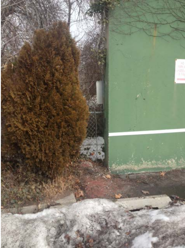
Existing sound wall along north property line
